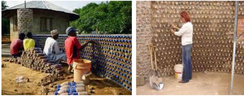
Fig. 1. Use of plastic bottles wastes in building (Katdare, 2011; Alvarado, 2010).
