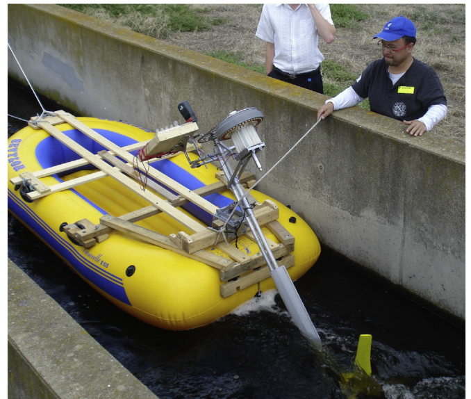
Fig. 6. Turbine and generator mounted on inflatable boat in Bolivar channel.
