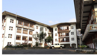
7 - reinforced concrete frame central government office building with brick infill walls
