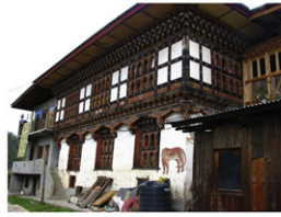
2 - contemporary rammed earth house with timber-frame rabsel
