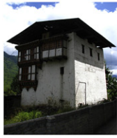
1 - rammed earth with timber-frame rabsel
