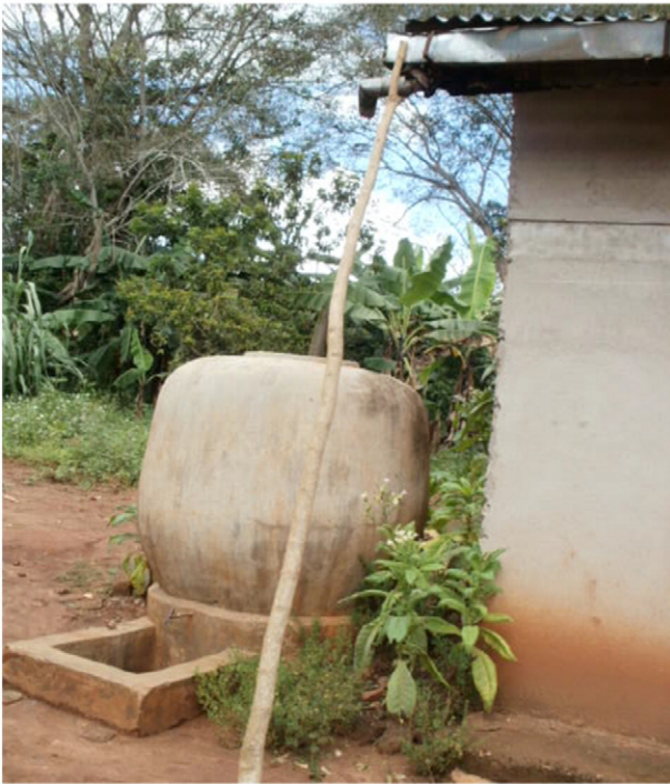
Fig. 4. Tank for rain water harvesting.
