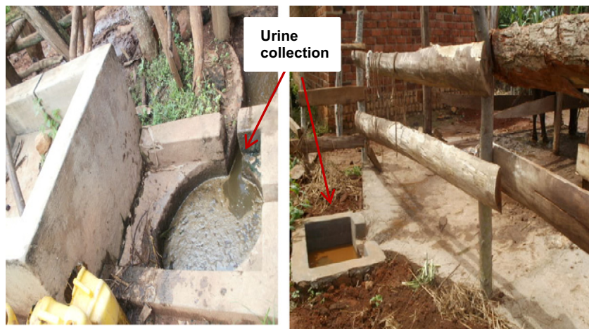
Fig. 3. Cattle sheds constructed with urine collection centers.
